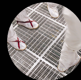
Purified air recirculates through ceiling and floor tiles.
